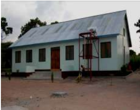
Volunteers Accommodation and Multipurpose Block
